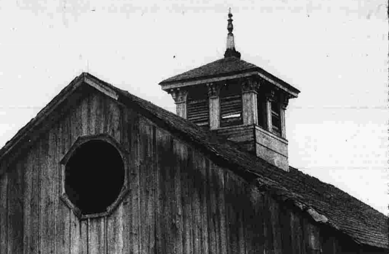
A Barn in Lebanon, Conn. (Photo by Doug Bevins)
